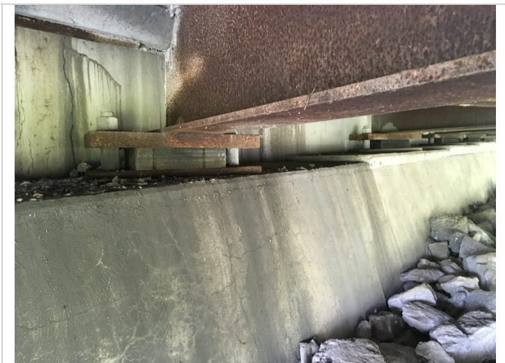
Bearing condition at abutment #2. Typical of all 10 at this location.
