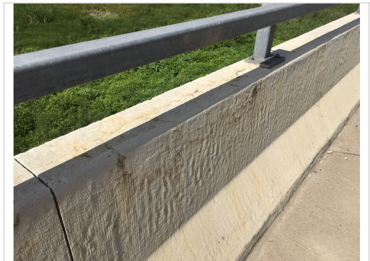
Map cracking in the bridge parapet. Typical of several locations.
