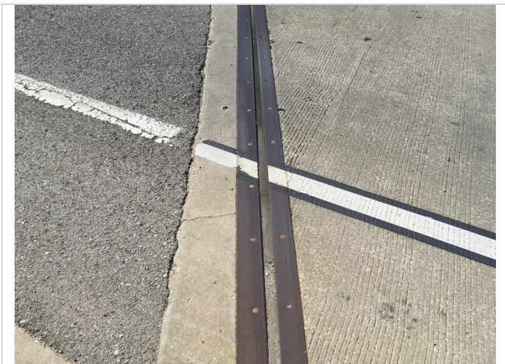
Typical joint seal condition at the abutments.
