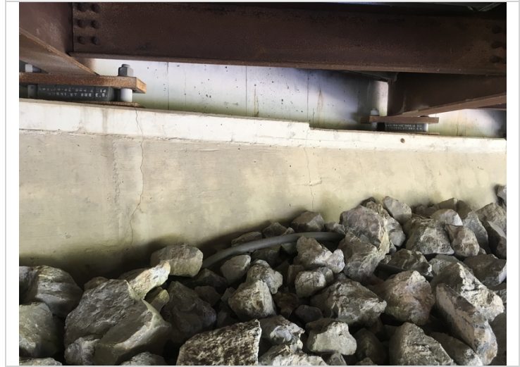
Cracking in the vertical face of the bridge seat in the original portion of the abutment.
