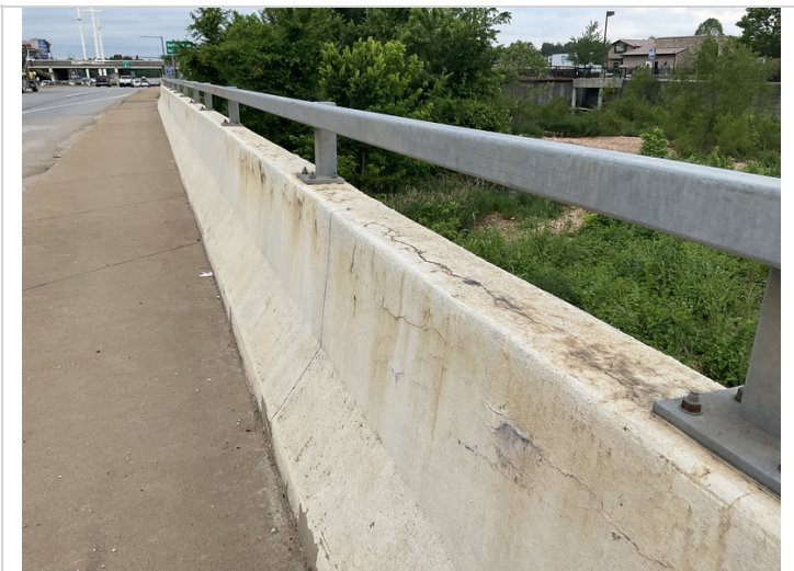
Cracking and delamination on top of parapet wall.
