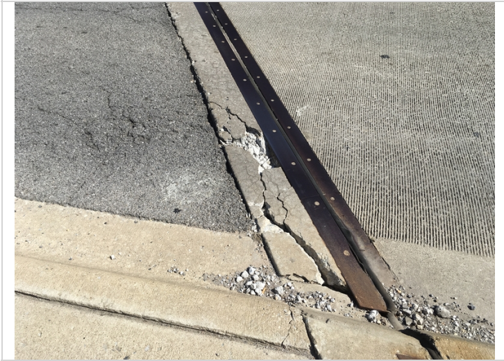
The top of the back wall at the left ending of the structure has deep spalling and is loose.
