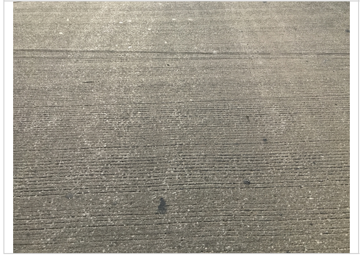
Typical longitudinal cracking in deck surface.
