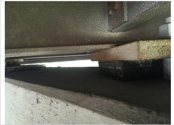
Bearing condition at bent #2. Typical of all 10.
