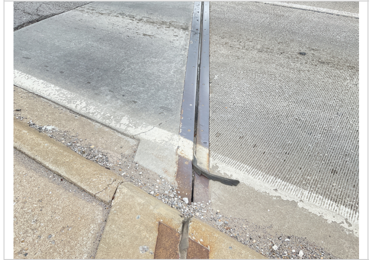
-The left side of abutment has approximately 3' of pourable joint material that has been displaced.
