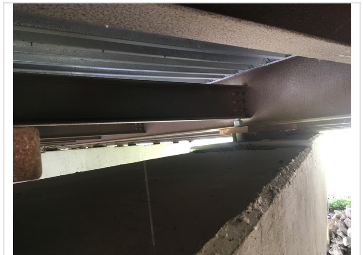
Bearing condition at bent #1. Typical of all 10.
