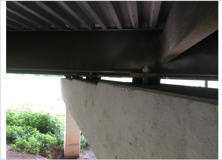
Bearing condition at bent #5. Typical of all 10 at this location.
