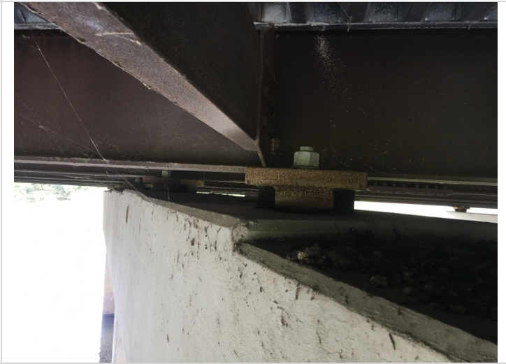
Bearing condition at bent #3. Typical of all 10.
