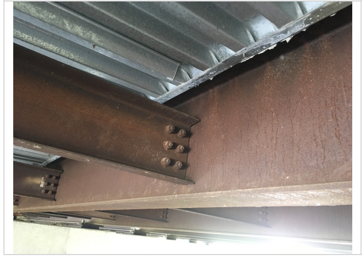
General condition of the weathering steel protective coating.
