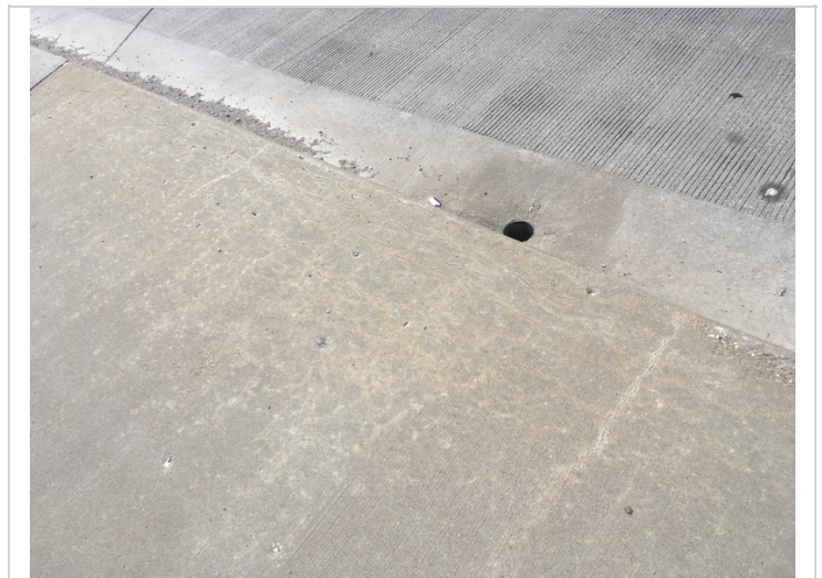
Map cracking in the edge of the right sidewalk over span #5.
