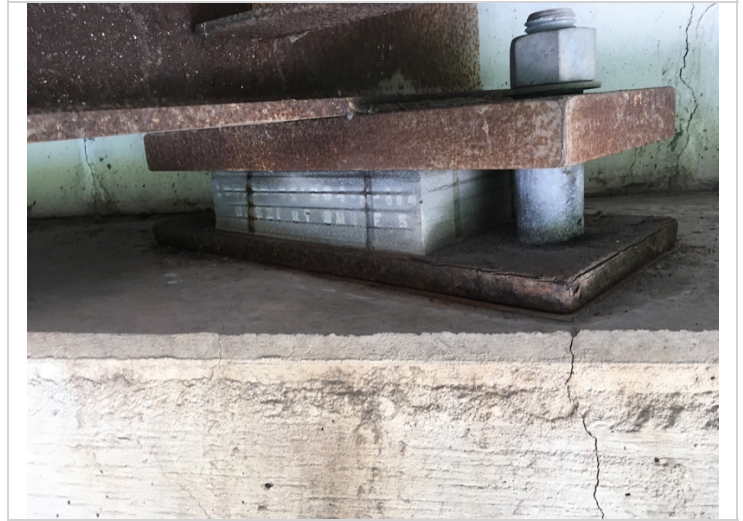
Bearing condition at abutment #1. Typical of all 10 at this location. Showing minor corrosion on the masonry plate.
