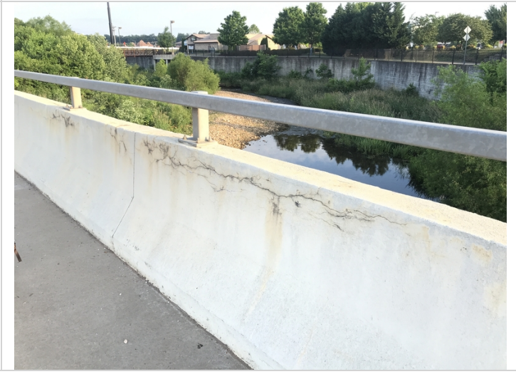
Horizontal cracking in the right parapet.
