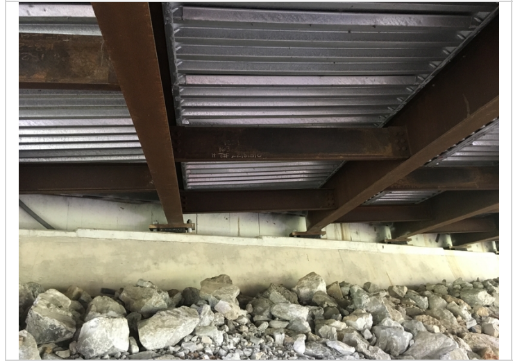
The beams are not centered on the bearings at abutment #2 at all the beams, the condition worsens as the beams continue to the right.
