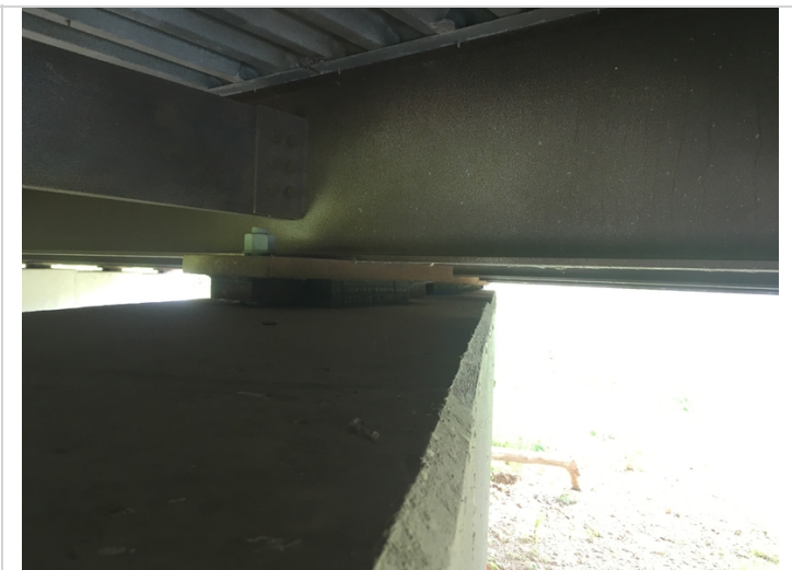
Bearing condition at bent #4. Typical of all 10 at this location.
